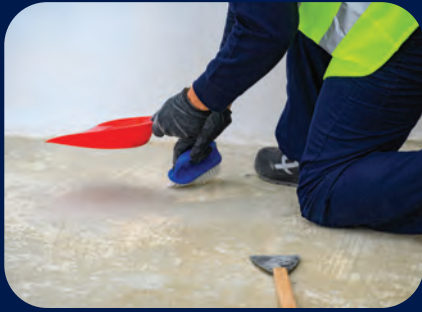
STEP 1 Preparation of the surface
