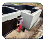
Foundations and retaining walls
