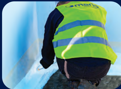
STEP 5 Wall-floor connection
