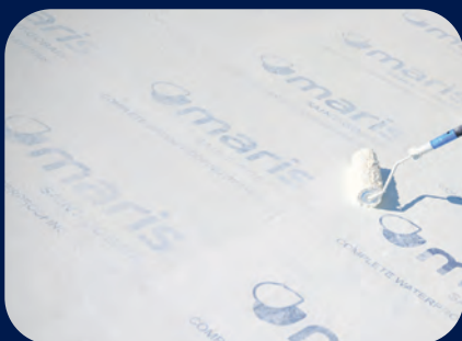
STEP 7 2nd layer of waterproofing membrane
