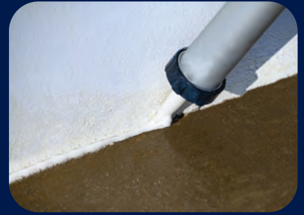
STEP 3 Fixing cracks and joints
