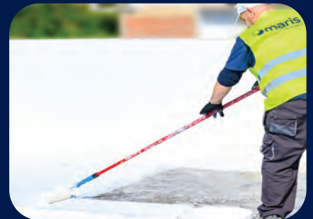
STEP 6 Reinforcement 1st layer of waterproofing membrane
